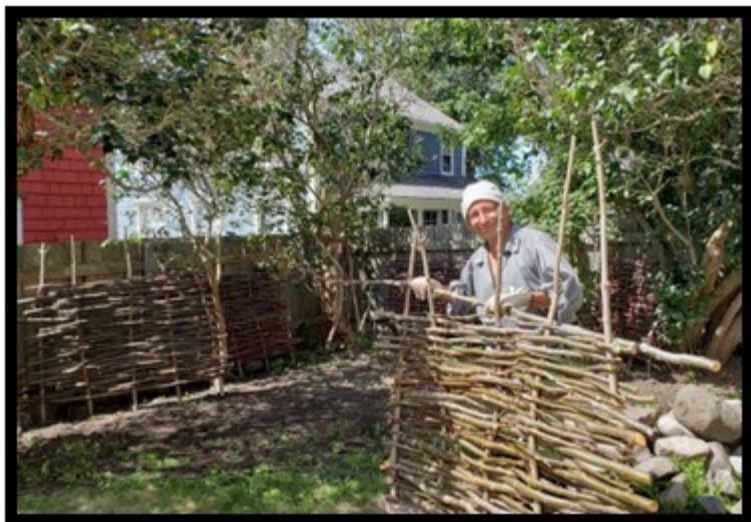
Above—Ross-Thomson House volunteer Rod Mossman preparing the walls for a chicken coop using wattle fencing
